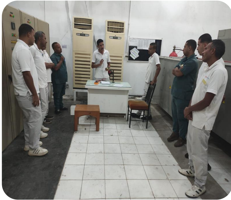
Figure: Engineering team technical briefing in the plant room. Monthly sessions cover energy management protocols and equipment maintenance procedures — directly supporting the resort's energy reduction targets.
