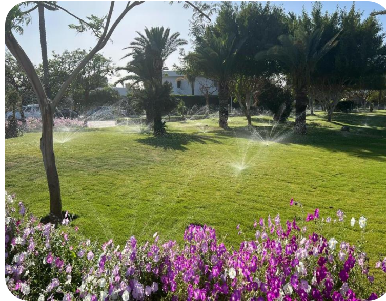
Figure: Automated irrigation across the resort's landscaped gardens. Schedules are timed to early morning hours to minimise evaporation losses in Hurghada's hot desert climate. The majority of irrigation demand is met from treated wastewater.
